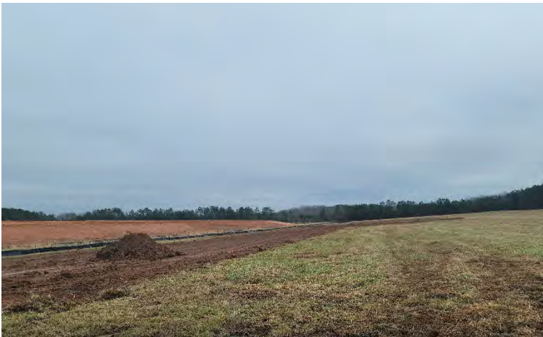
LF4-02: Some areas of subsidence were observed to be holding water. Repairs are being address during the cap and closure activities currently underway.
